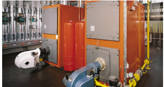
Gas inlet pressure monitoring on high-performance boilers
